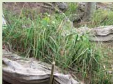
Eco-logs in 2007 which have begun to decompose and collect sediments and organic material
