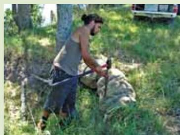
The eco-logs are secured using wooden stakes and shaped into arcs to create a pooling effect which then overflows to the next pool
